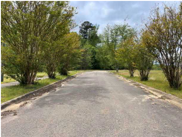
Photo 3 Paved roadway onsite
