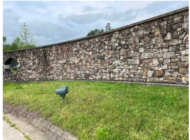
Photo 2 Rock wall on east side of site
