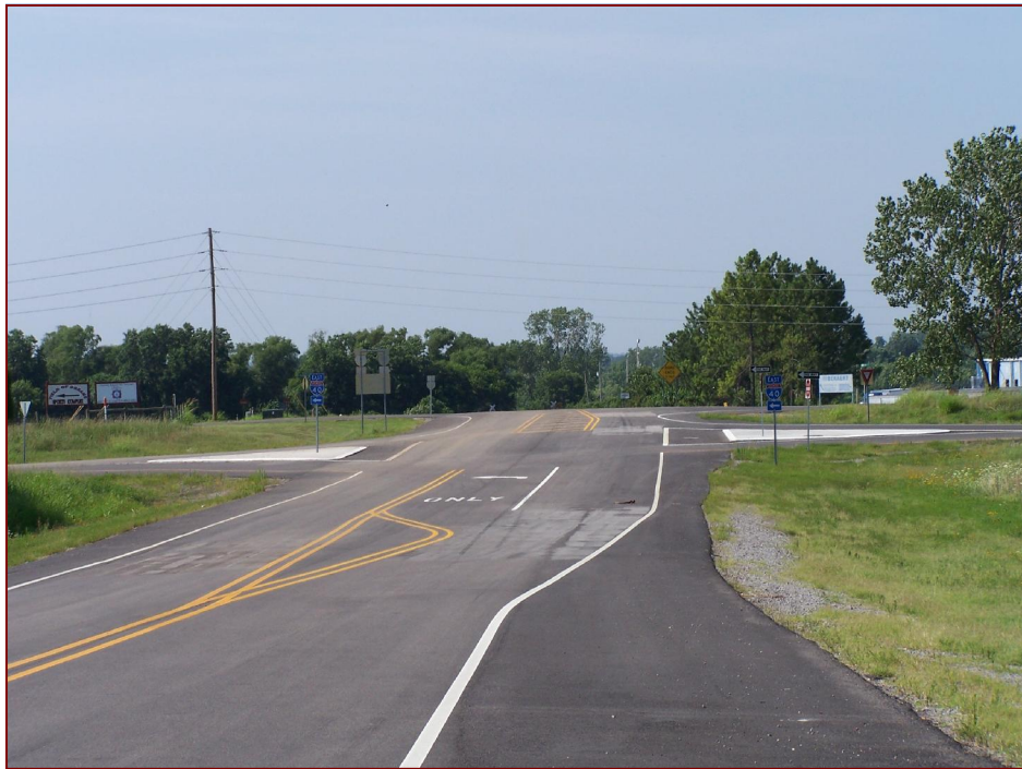
Looking South towards Bluff View (photo taken from the Interstate Overpass)
