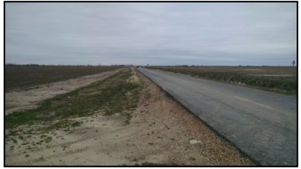
32 : Arkansas Highway 119 bisecting the northern 1/2 of the Subject Property (facing west)
