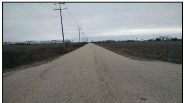
30 : Denso Road providing ingress/egress to the southeast corner of the Subject Property
