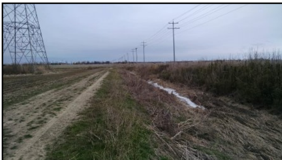
23 : Electrical service lines running parallel to the un-named ditch bisecting the Subject Property (east-west)
