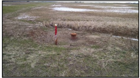
14 : Irrigation riser associated with agricultural wells on the Subject Property
