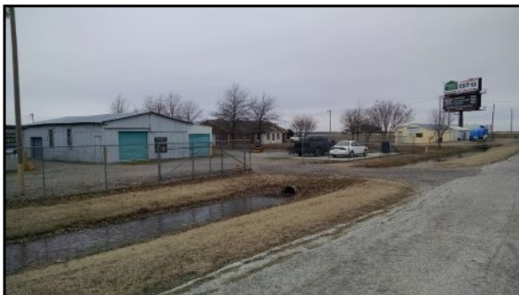
11 : Commercial facility & office (storage facility) as well as single-family residence located in the northwest corner of the Subject Property
