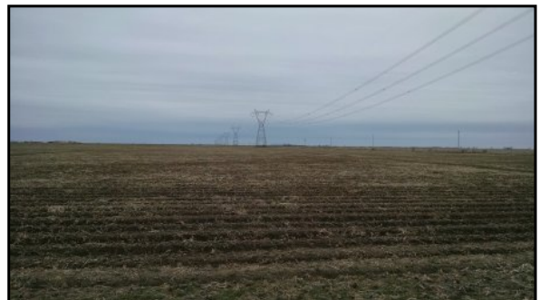
24 : High-tension transmission line running along the eastern edge of the Subject Property (facing north)
