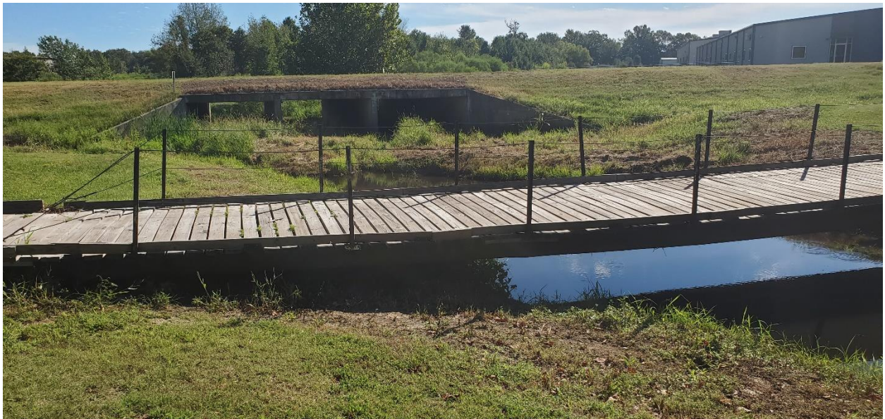
Perennial stream exiting sports complex and the Queensway St. box culvert
