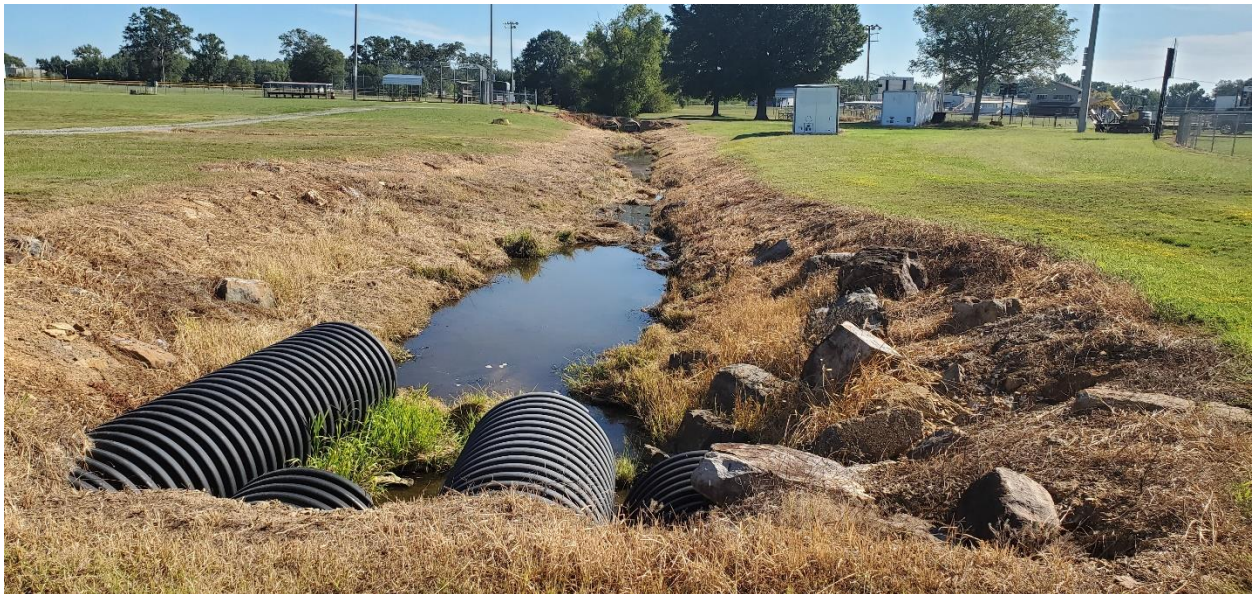
Perennial stream entering west side of the complex through pipe culverts
