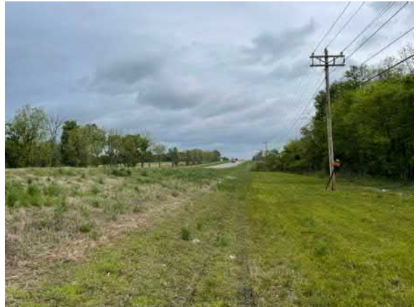
Photo 12 Power lines on western site boundary
