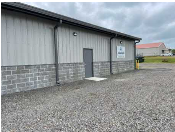
Photo 5 East adjacent City of Arkadelphia office/storage building
