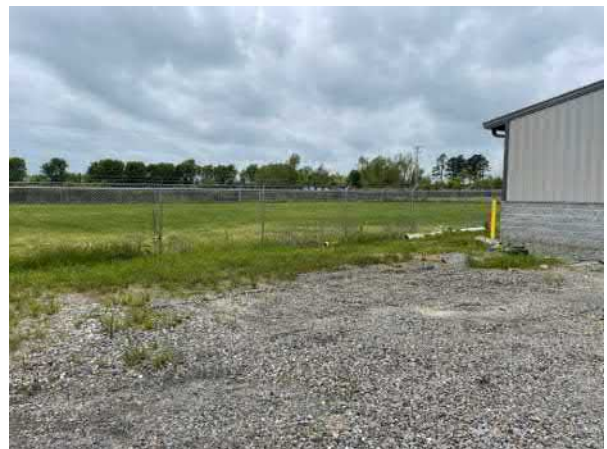
Photo 6 Fenced area for east adjacent building
