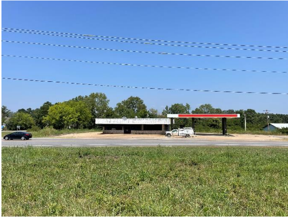
Photo 7 Closed gas station adjacent to the north
