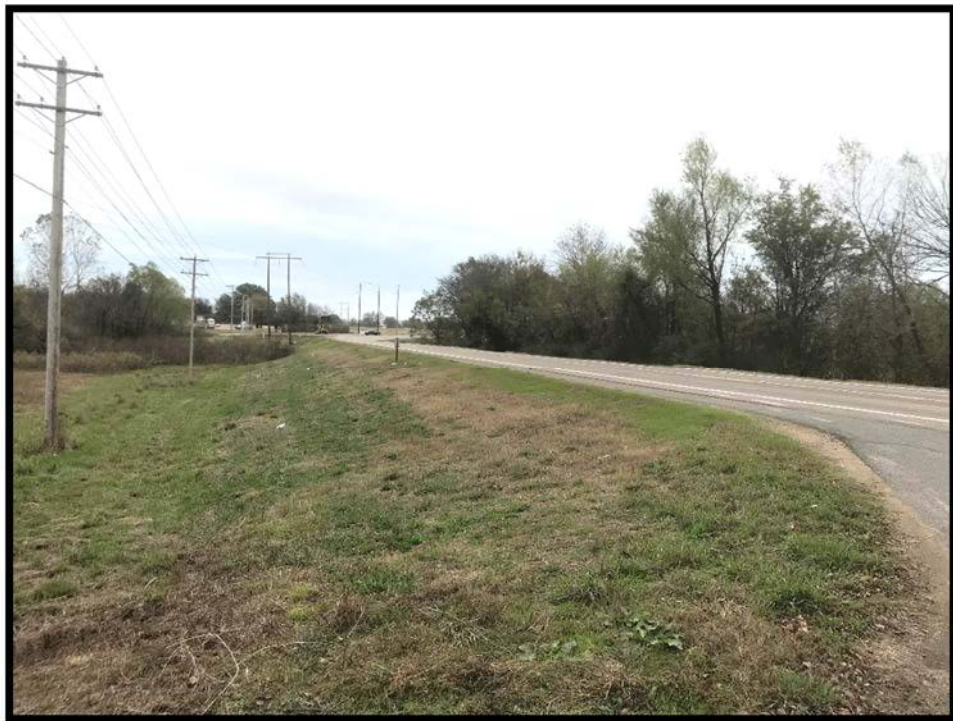
Photo #18 View looking east down State Highway 32 N.
