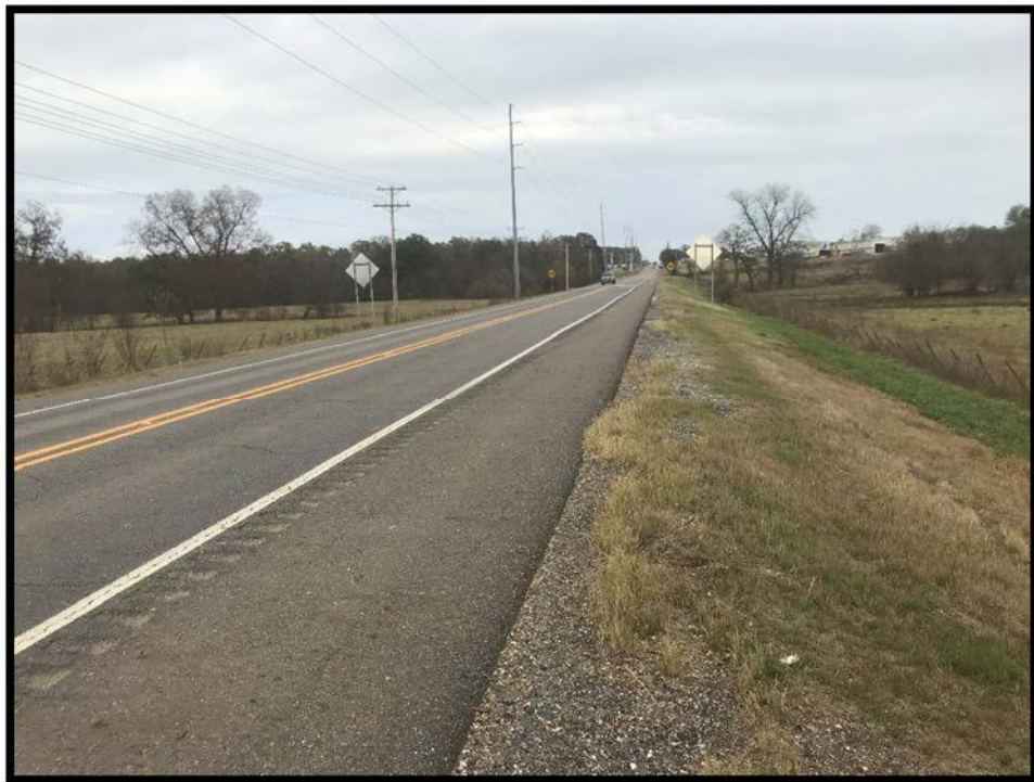
Photo #4 Looking east down State Highway 32 N.
