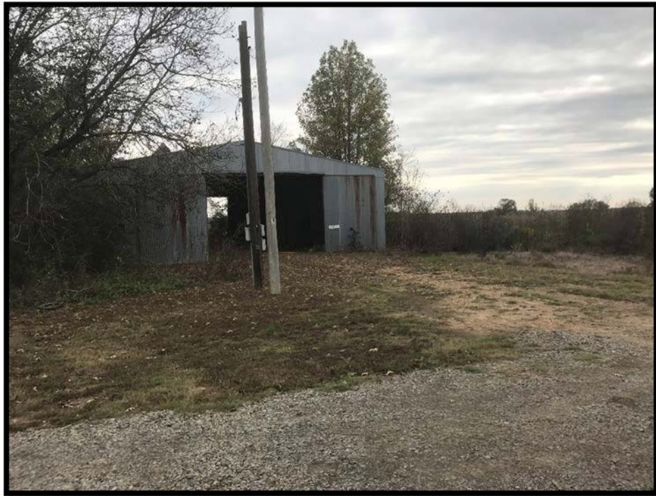
Photo #13 Dilapidated barn located on 162 acre lot.
