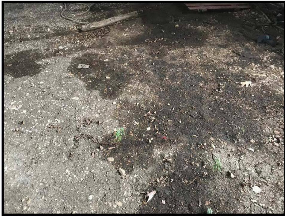
Photo #15 Interior and staining in dilapidated barn located on 162 acre lot.
