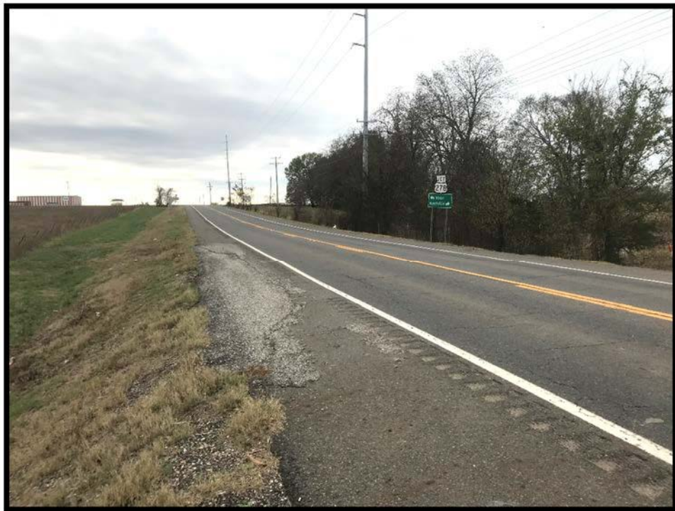
Photo #2 Looking west up State Highway 32 N.
