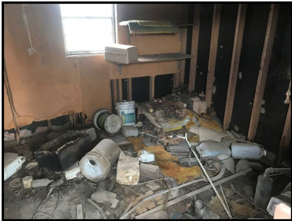
Photo #16 Interior of old well house located on 162 acre lot.
