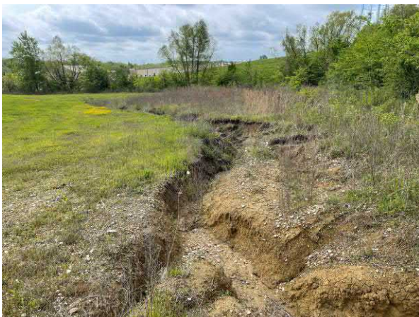
Photo 5 Drainage on western portion of site
