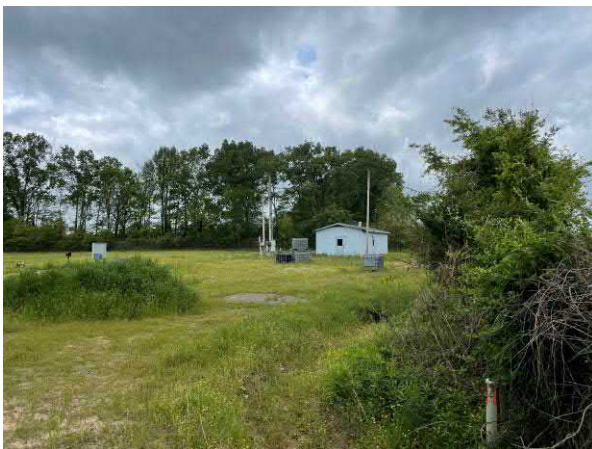
Photo 15 South sewer lift station
