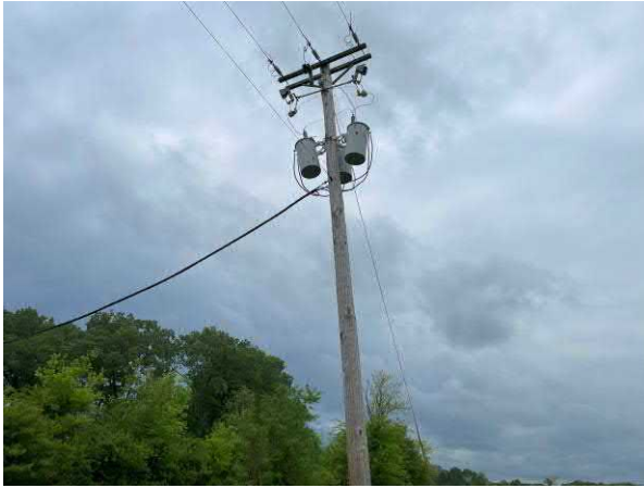
Photo 7 Pole-mounted transformer on south site boundary
