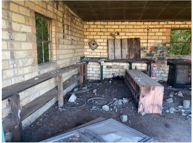
Photo 8: View former tool shed in northern adjacent storage building.
