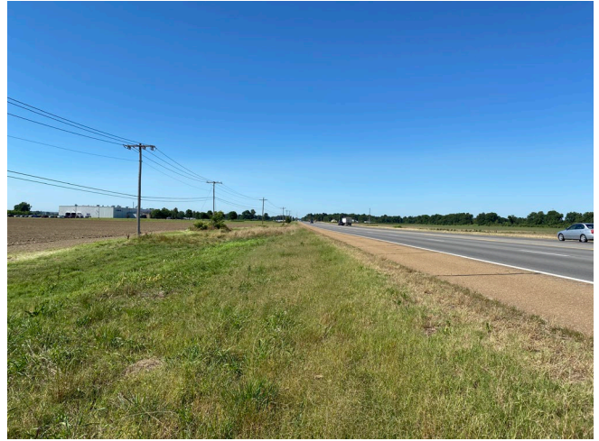
Photo 2: View along S. Falls Blvd looking south.
